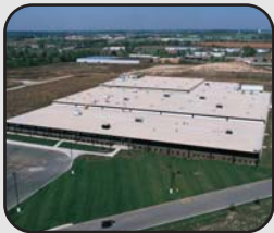
Orland Park, Illinois, USA
